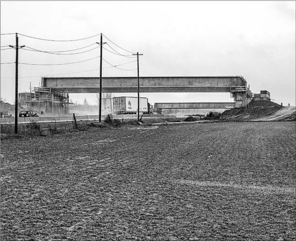
Dilon Rosseau photo The concrete bridge slabs for the 407 Highway were recently installed over Highway 115/35, the end point of the new highway. The photo was taken from the south side of the overpasses.
